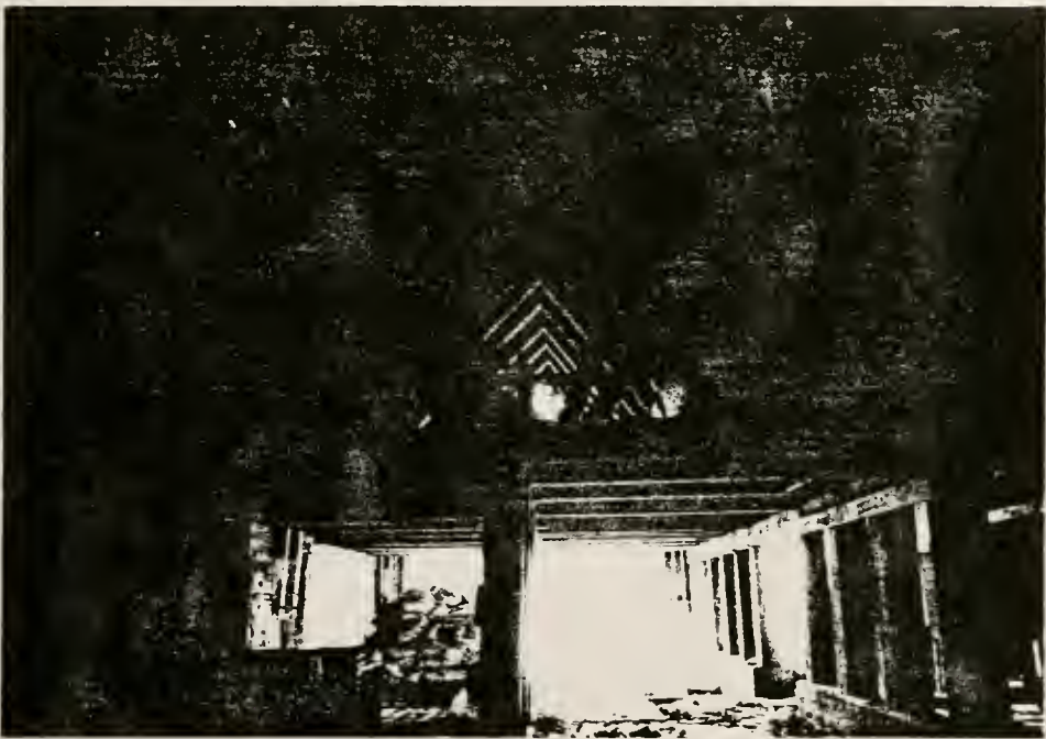
Figure 97. Revenue Mill (structure #34) interior of upper level, looking south at the timber substructure of the new ore bins.
